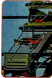
Deck Link w/Steel Barriers
